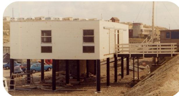
Built on a tight budget with members' donations, the predicted lifespan was just 25 years. The simple yet strong design greatly exceeded these expectations, and lasted for 50 years! But with decades of exposure to the natural elements, the steel structure of the building ultimately corroded, and the building had to be closed in late 2023.
